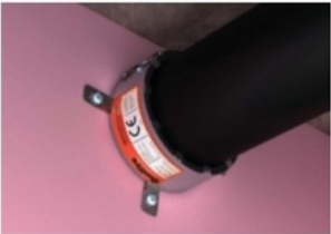
Fire collar fitted to wall
