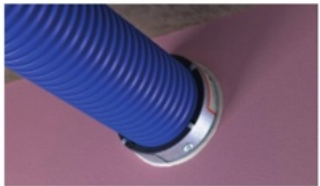
Fire collar fitted to wall
