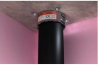
Fire collar fitted to ceiling/floor
