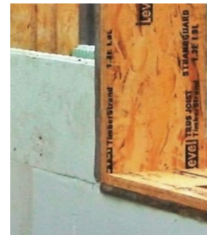
ICF (Insulated Concrete Form)
