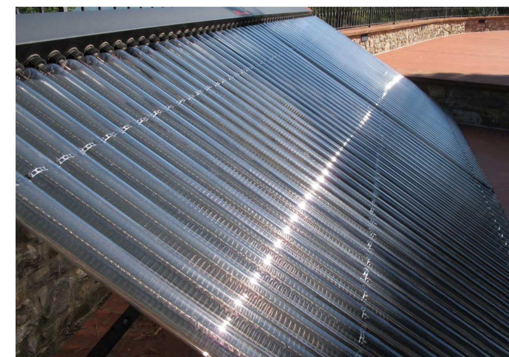
Bottom: Solar Thermal Panels
