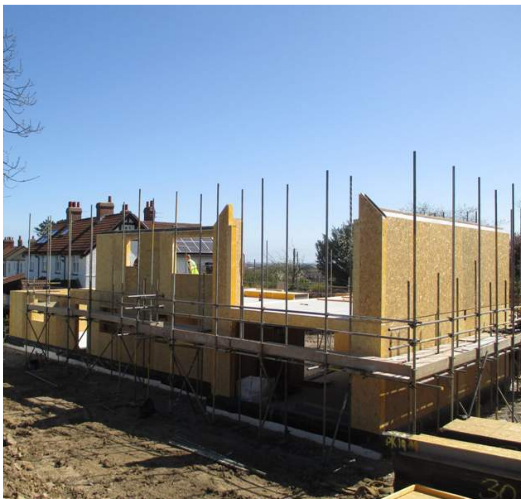
Top: SIPs, Panel Construction Bottom: Laying Foundations
