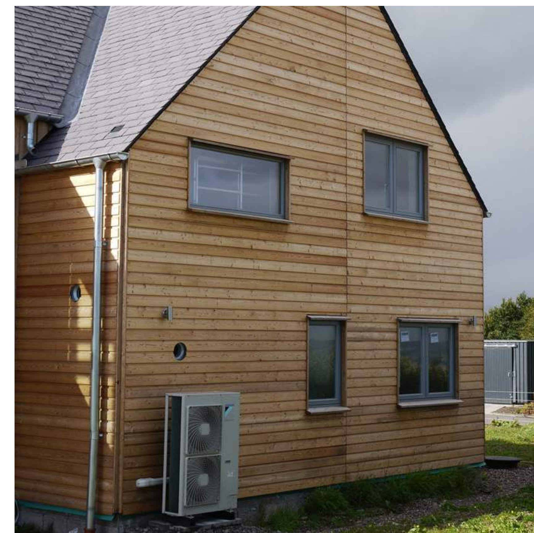
Bottom: Air Source Heat Pump
