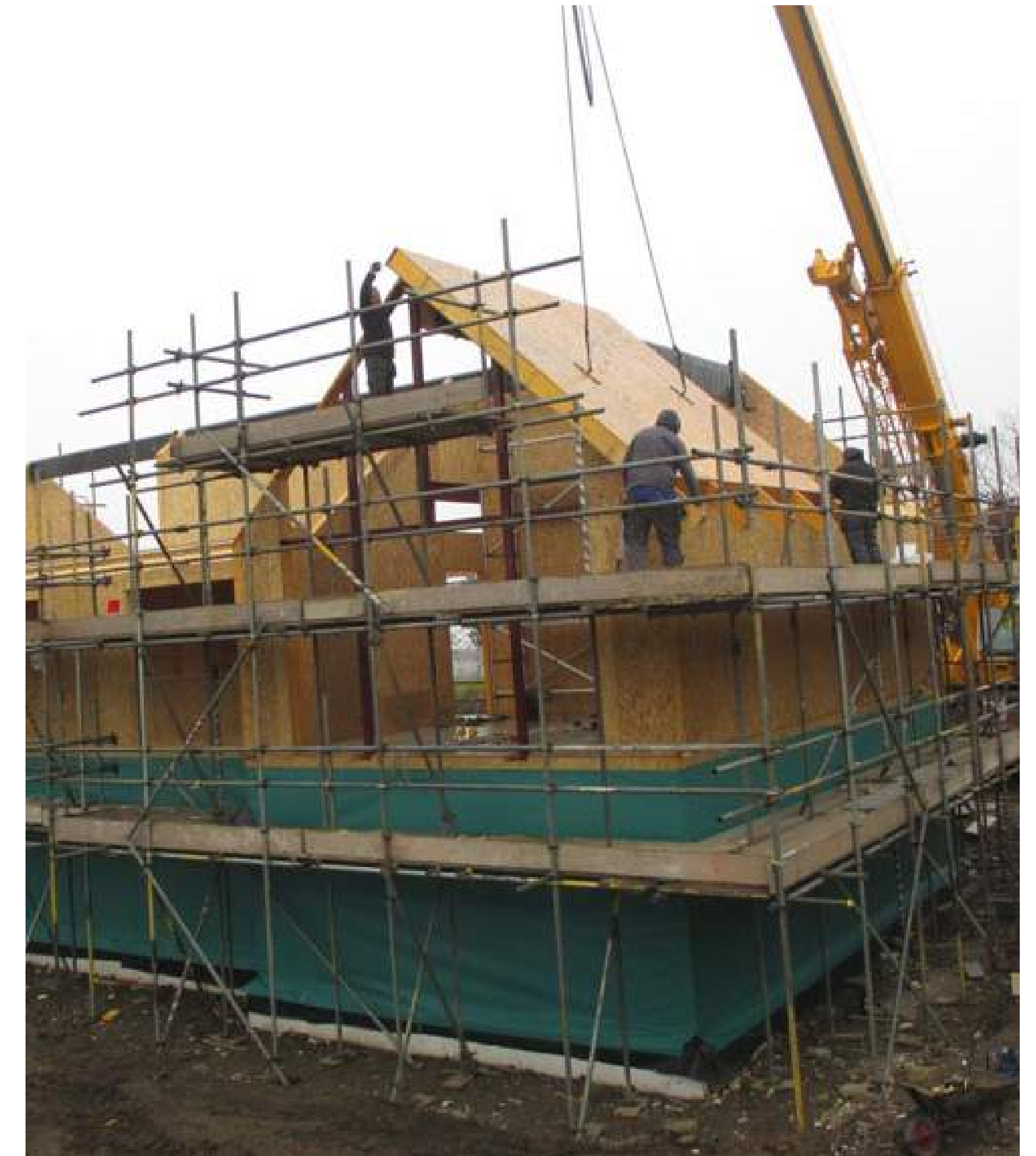
Top: SIPs Roof Goes On
