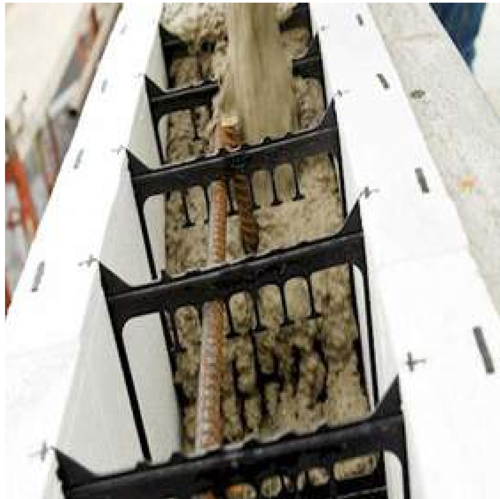
Top: Insulated Concrete Formwork Pour Below: Cross Laminated Timber Home Build
